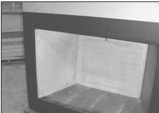
Figure 8.6 Side Refractory Installed
